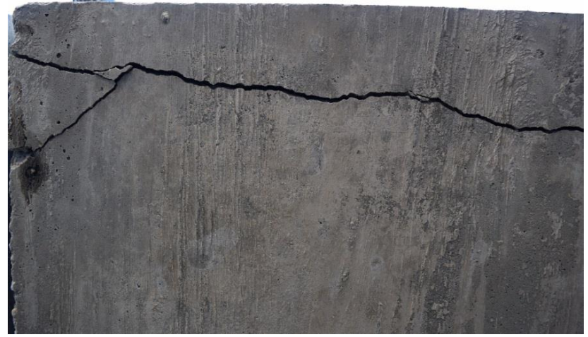
Bottom of deck, downstream of joint
