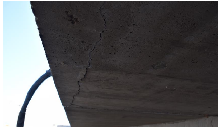
Bottom of deck, downstream of joint
